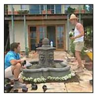
Water feature: When laying a pre-made water feature, create a level base using roadbase or a dry bed of concrete (screeded and set) or on a bed of paving sand. Low voltage and low voltage transformer was run to the pump for added safety.
